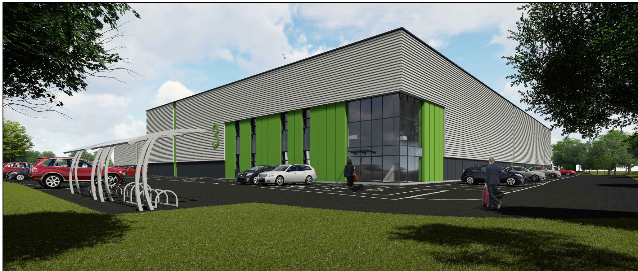
View North East - Unit 3 Office Entrance
